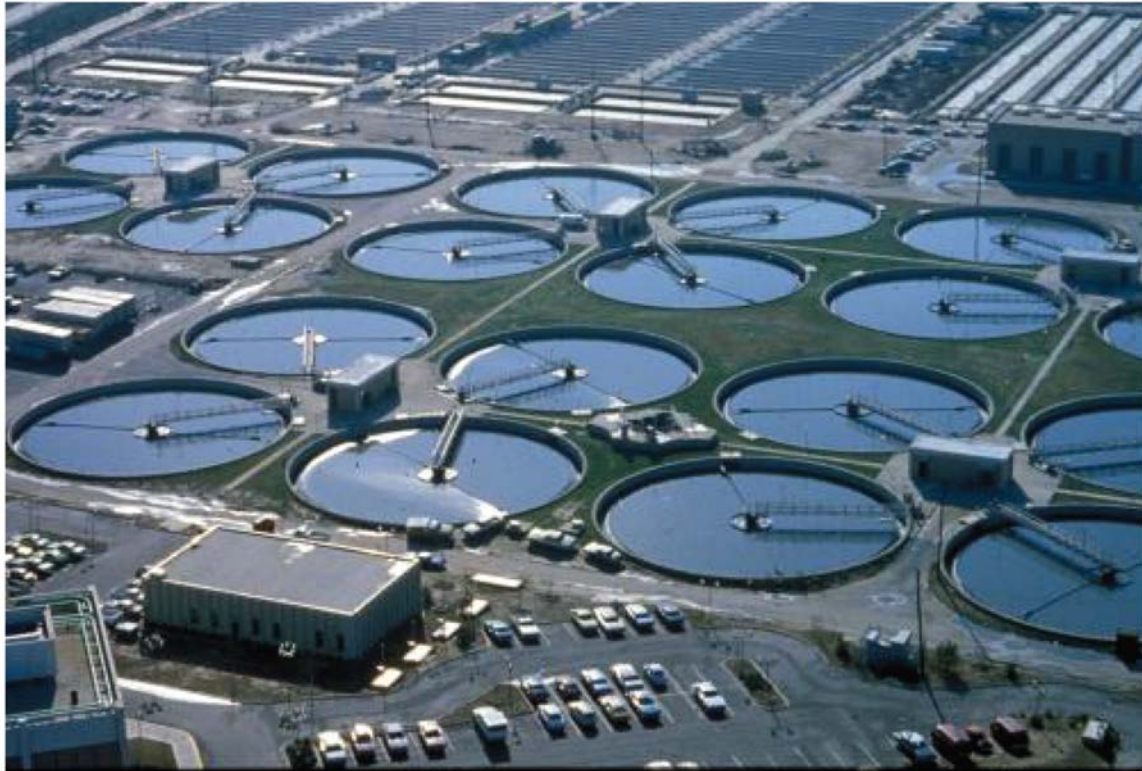
Figure 25.1 Sewage Treatment Plant (credit: "eutrophication&hypoxia"/flickr.com)
